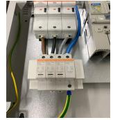
Connect from the Neutral terminal of the SPD up to the Neutral Bar. Tighten the connections from the Fuse Carrier to the Top of the SPD.
