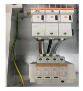
Fit the Fuse carrier on the top Din-Rail next to the Incomer. Fit the SPD and Blanks either side of the SPD on the Din-Rail below.
