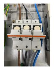
Fit the 125A 22x58mm Fuses provided in the 3 pole Fuse Holder.
