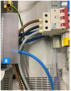
Connect the top of the Fuse Carriers to the Main switch using the cables provided.
