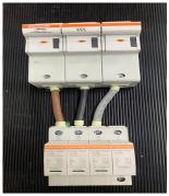
Short cables must be fitted first before fitting onto the DIN rail. Brown wire: L1 SPD to L1 Fuse Holder. Black wire: L2 SPD to L2 Fuse Holder. Grey wire: L3 SPD to L3 Fuse Holder.
