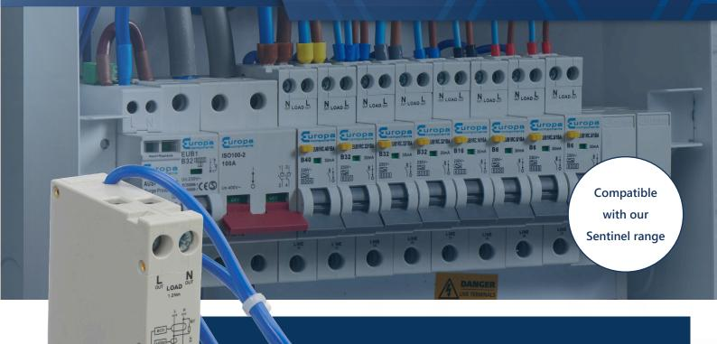
Our AFDDs come with an incorporated Type A RCBO for enhanced protection
