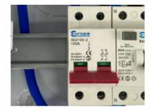
1) Create 2 additional module spaces by sliding the main switch, RCCB and MCBs to the right.
