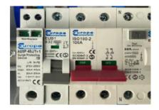
2) Insert the SPD to the far left side and the 32A Type B MCB in between the SPD and main switch.
